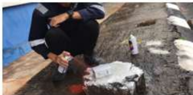
Rajah 4: Gambar spray besi
